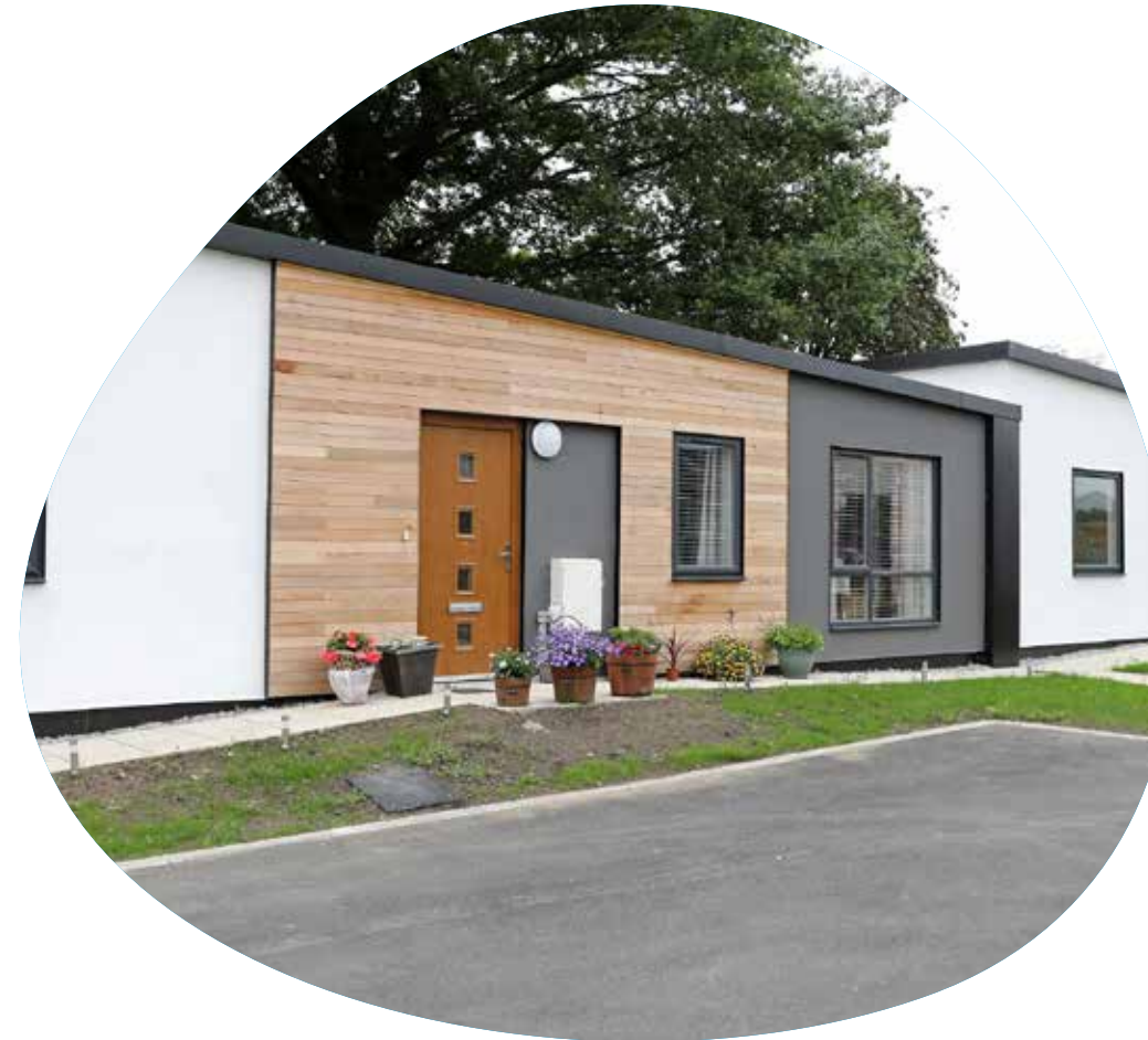
Off-site volumetric construction (HUSK) Parkside, Stanley
