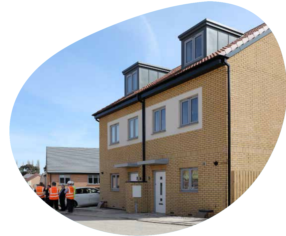
Off-site volumetric construction (Ilke) Central Park, Darlington
