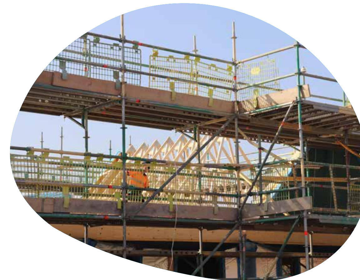
Timber frame construction Field Lane, Selby
