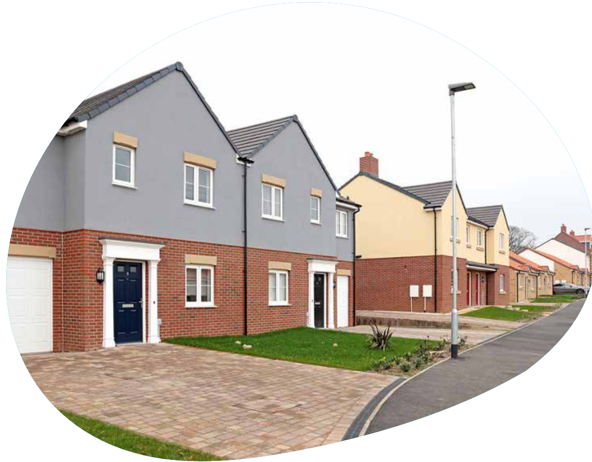
Insulated concrete formwork (ICF) Station Manor, Hartlepool
