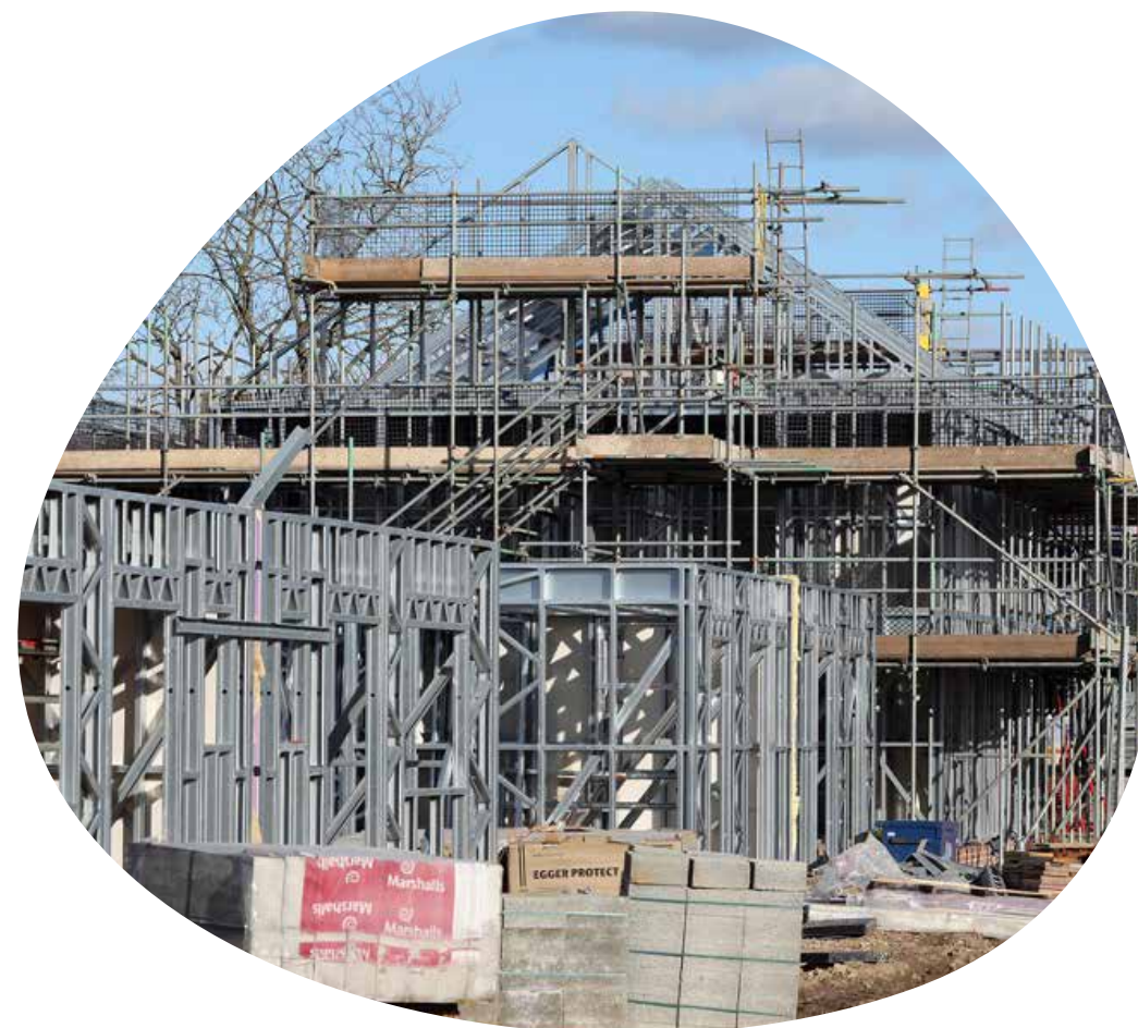
Light Gauge Steel College Grange, Sunderland
